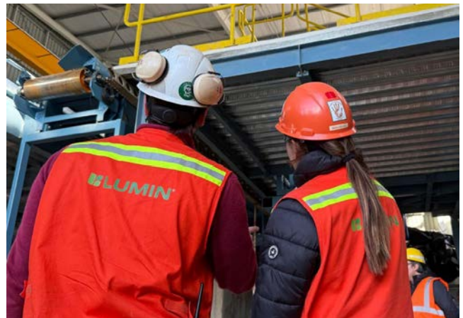
Construction of Lumin's Melo mill underway | Image credit: Lumin
